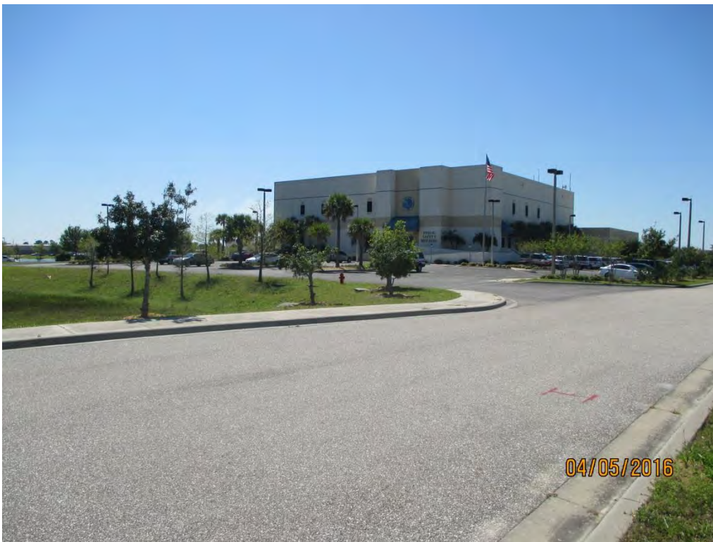
View to the southeast from Airport Road of Charlotte County Public Safety Building
