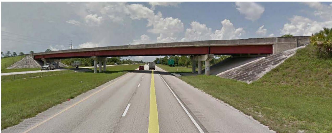
Figure 8-12: Elevation View of S. Jones Loop Road Bridge over I-75 (Looking North)
