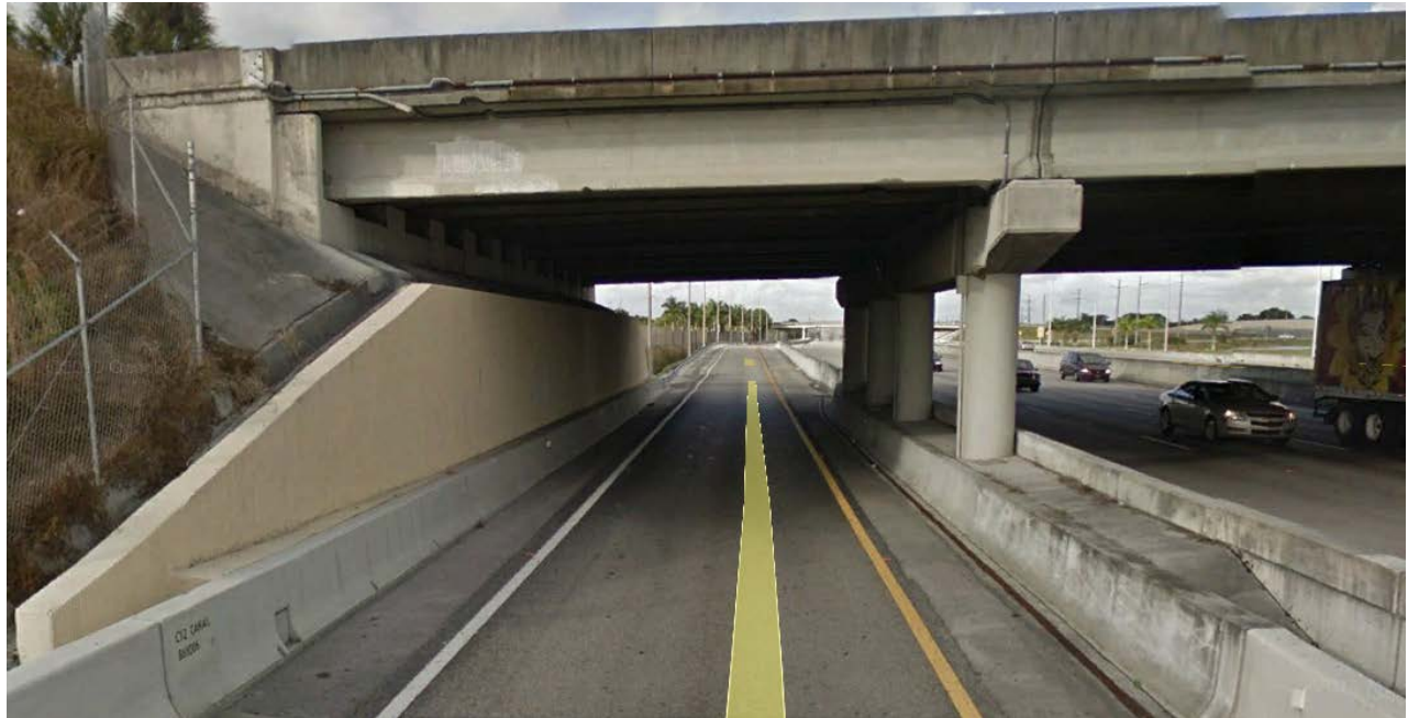
Figure 8-10: Photograph of Typical Tied Back Bridge Abutment Wall
